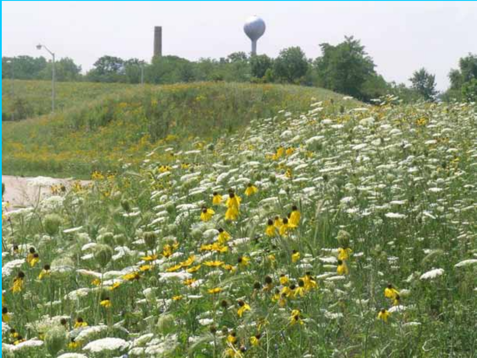
North Side Water Reclamation Plant
