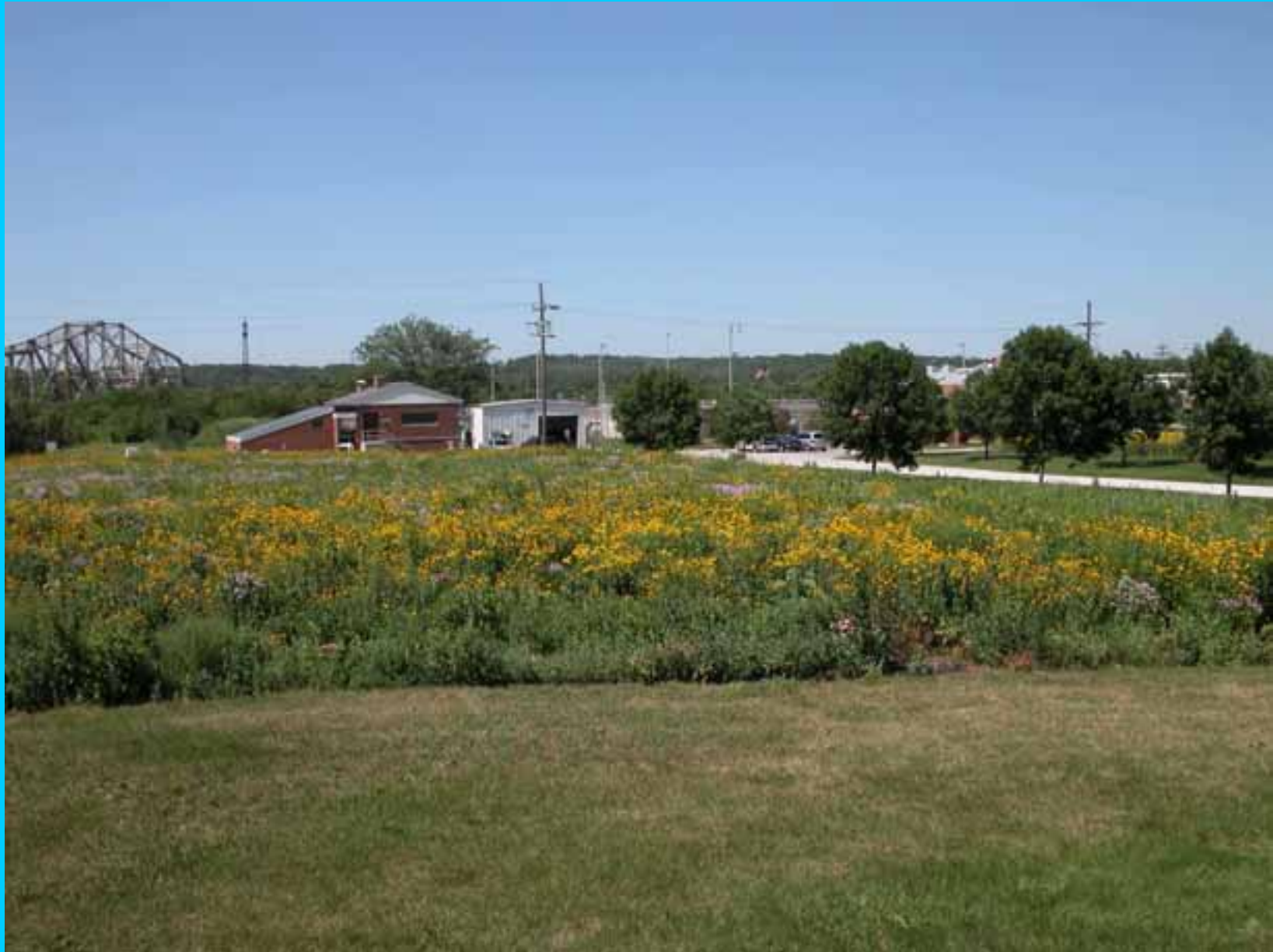
Lemont Water Reclamation Plant
