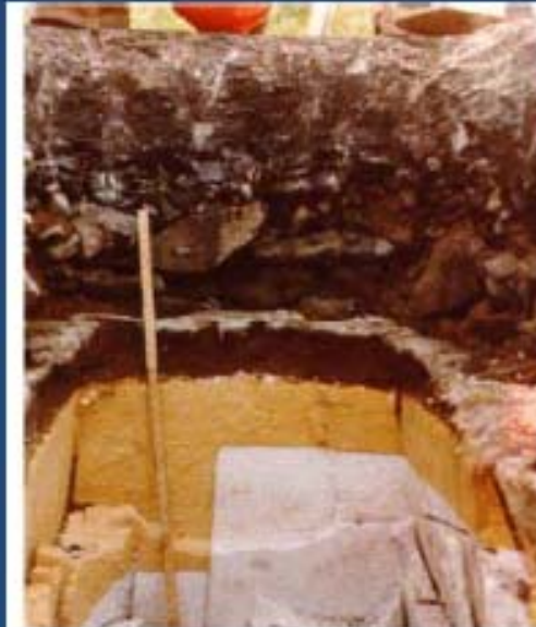
Figure 3. Excavation of the first EPS embankment at Flom bridge (EPS and polyurethane as protective layer).
